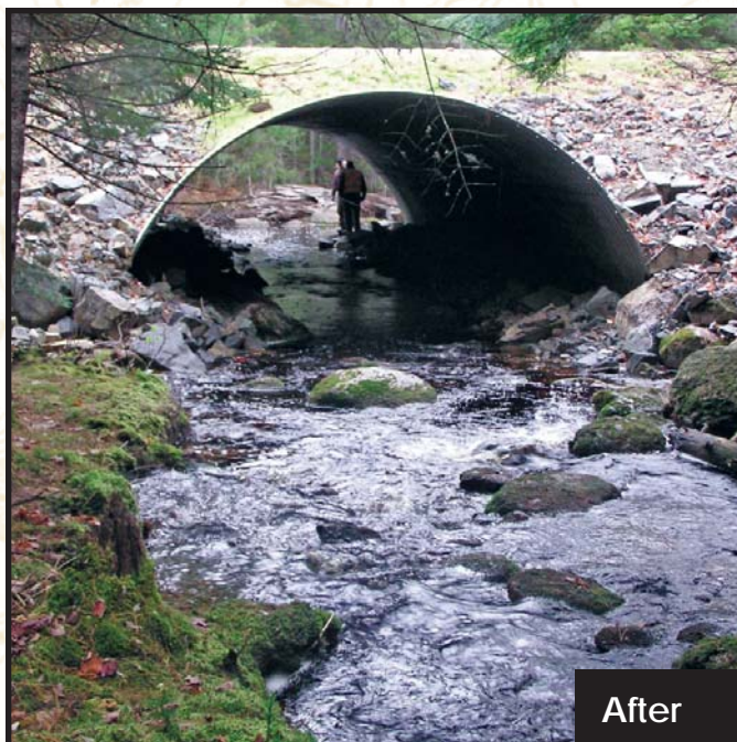
The much wider open-bottom arch that replaced the undersized round culvert allows salmon and trout to pass year-round. Open-bottom arch culverts simulate the natural stream channel.
